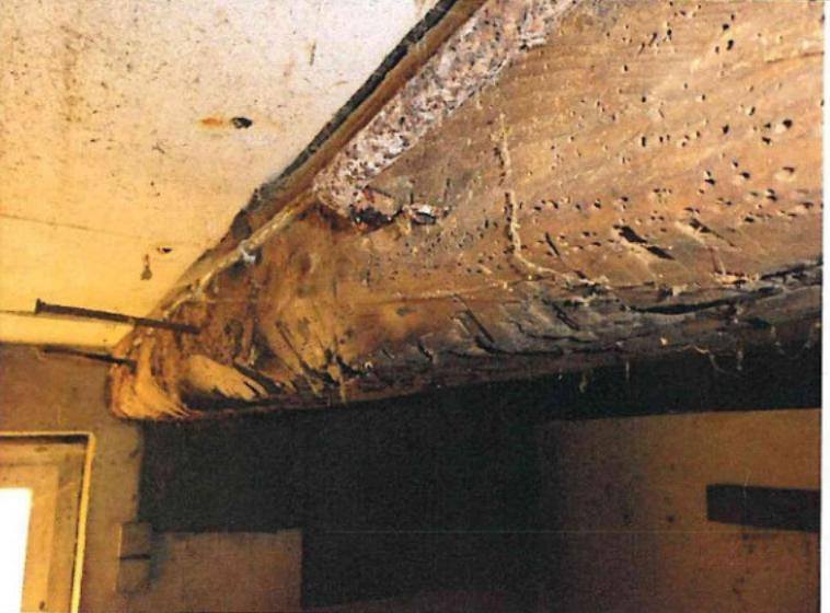
A close-up photograph of a basement ceiling. The surface is heavily perforated with numerous small, dark holes, characteristic of wood-boring insect infestation (Hausbock). The wood is discolored and shows signs of significant damage.                                             |
