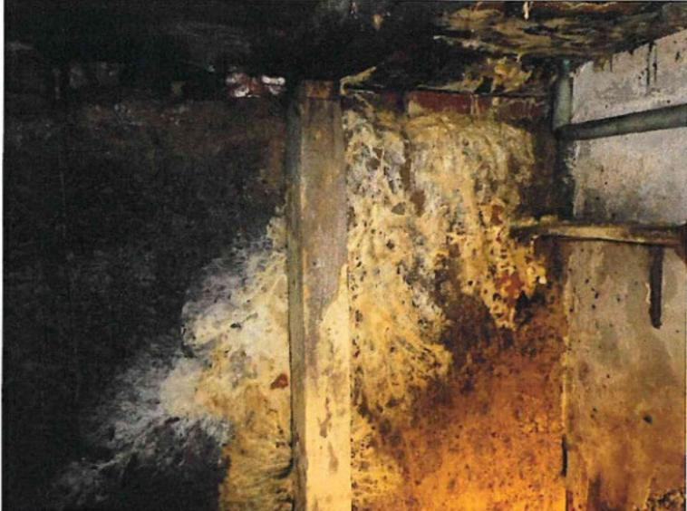
A photograph showing the interior of a basement. The ceiling and walls are heavily damaged, with large areas of white and yellow mold growth. The wooden structure of the ceiling is exposed and appears to be rotting. The lighting is dim, highlighting the extent of the infestation. |
